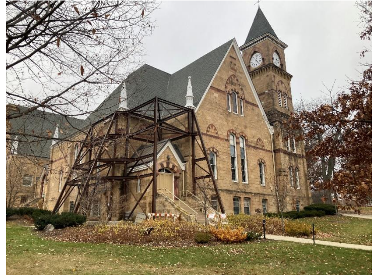
Structural supports (southeast corner)
