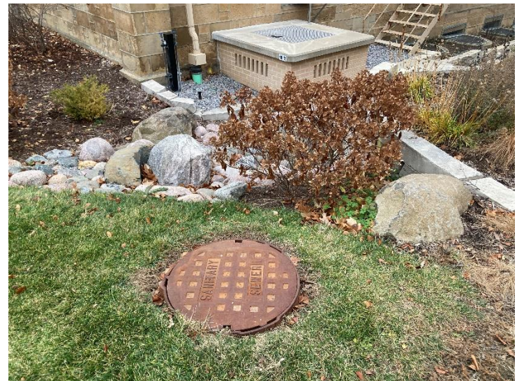
Sanitary sewer manhole
